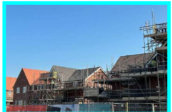
First homes under construction
