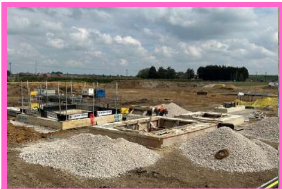
Pump Station 2—progressing well
