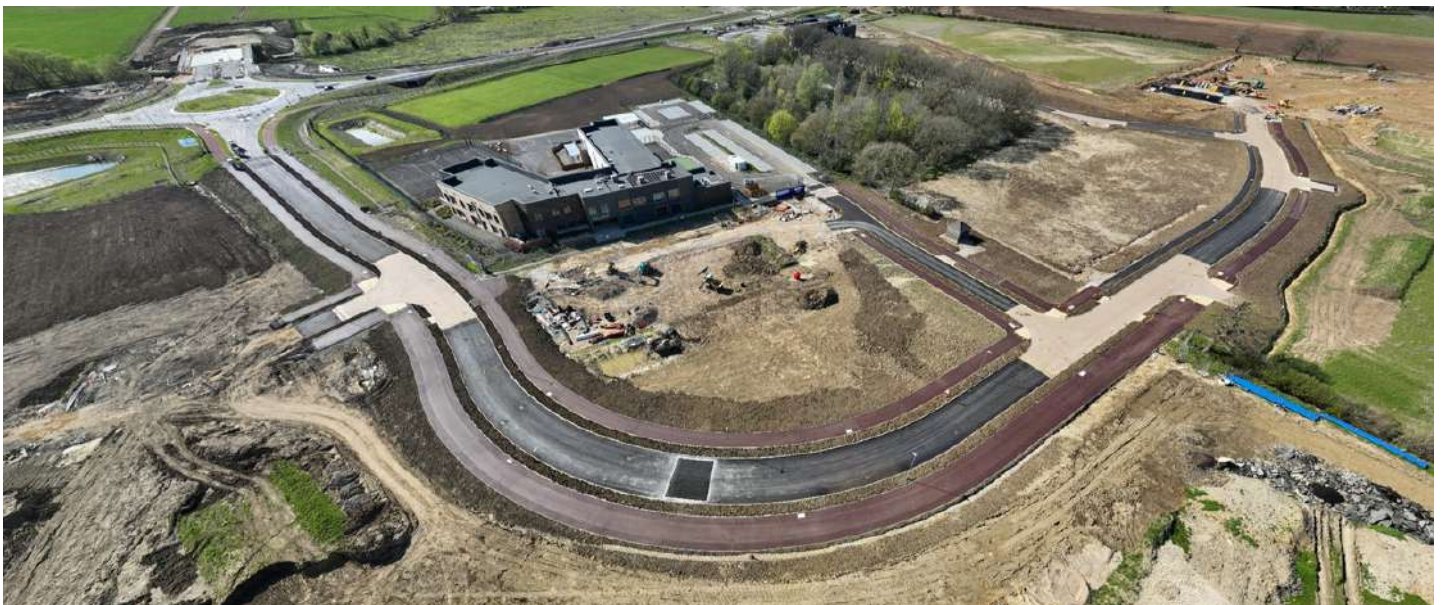
Primary Street 1 South extent of works
